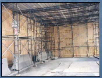
> Make a hoe ram disappear! Needed to work all night long near residential area > Built the "Flynn Memorial Garage" > Three-sided, roofed enclosure > Double-layer plywood walls Insulated wall air gap Successfully reduced hoe ram
