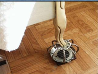
Annoying building vibrations Unexpected problem Caused by shifting elevated I-93 Artery onto temporary columns Significant community outrage > People could not sleep Complained of a variety of maladies Politicians and media got involved Extensive vibration study done Confirmed disturbing vibration levels > Vibration control measures Scarify/smooth Artery surface Install vibration isolation bed springs
