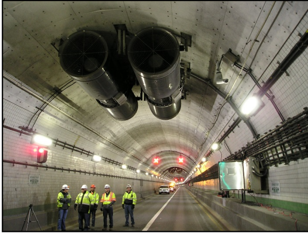
Photo 1. Approx. Midpoint DTWB Tunnel
