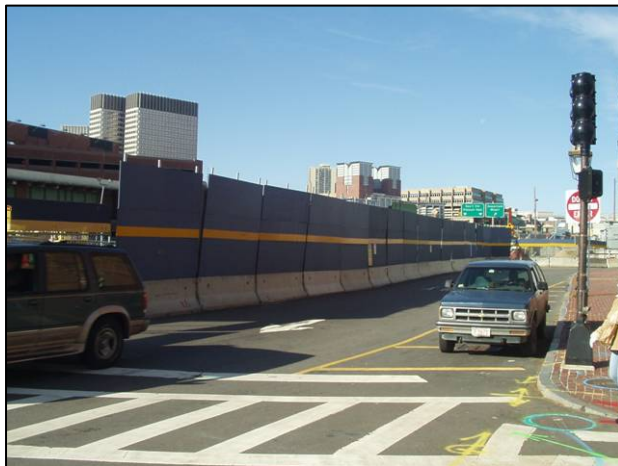
Photo 1. Plywood Barriers on Jersey Bases
