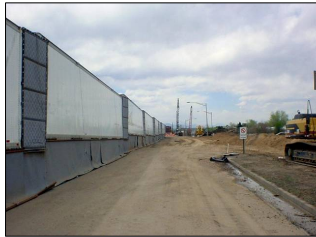
Photo 2. Container Trailers as Noise Barrier
