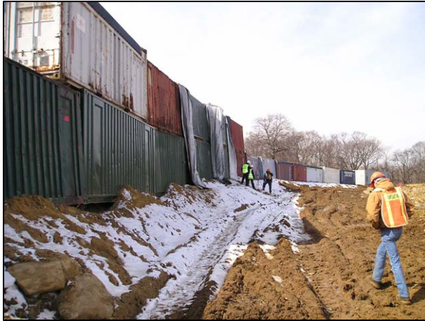
Photo 5. Conex Boxes used as Noise Barrier
